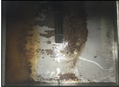
Figures 12a & 12b. Interior of the Wet Gas lube oil reservoir before cleaning (left) and post cleaning (right).
